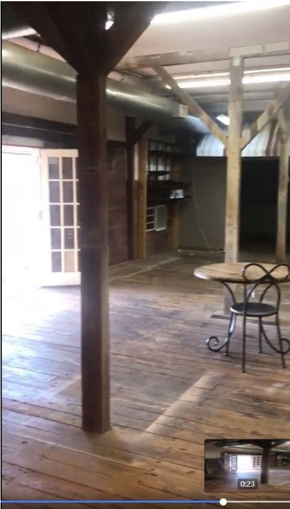
A glimpse of the interior under construction at The Line.
